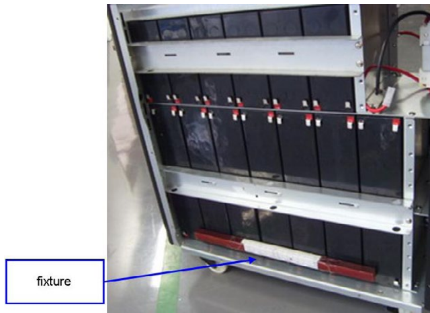
EBP40 with 40 Batteries Installed
