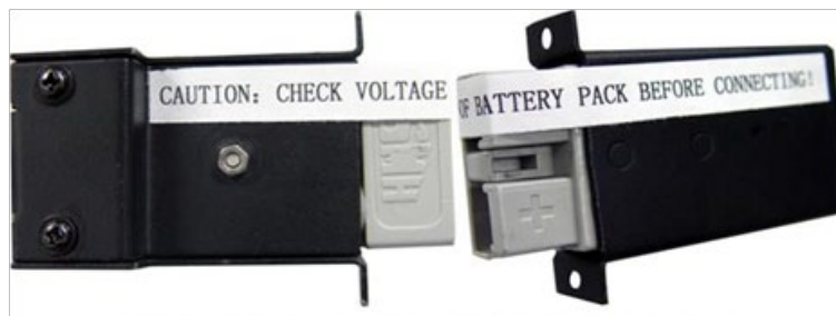
Caution label on CBP cable connectors - PLEASE CHECK VOLTAGES CAREFULLY
